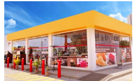
FUEL STATION BUILDINGS
